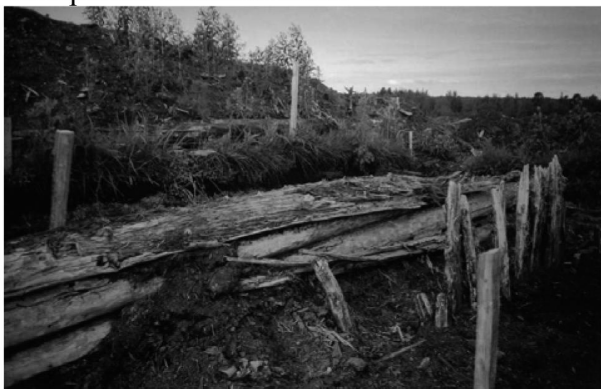
Завалинка постройки 6. Obstruct of construction 6
